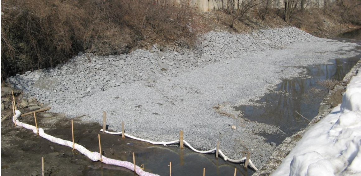
Completed Cap with Armor and rip rap on slope
