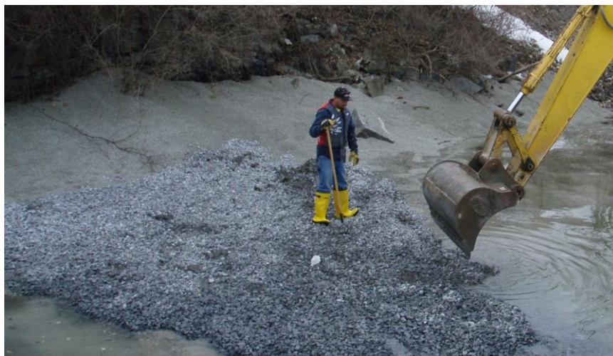
Placement of stone armor over AquaBlok low permeability capping material
