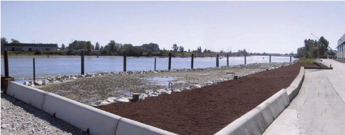
Photo #4: View of Completed Marshland, Riparian Zone, and Wharf Area
