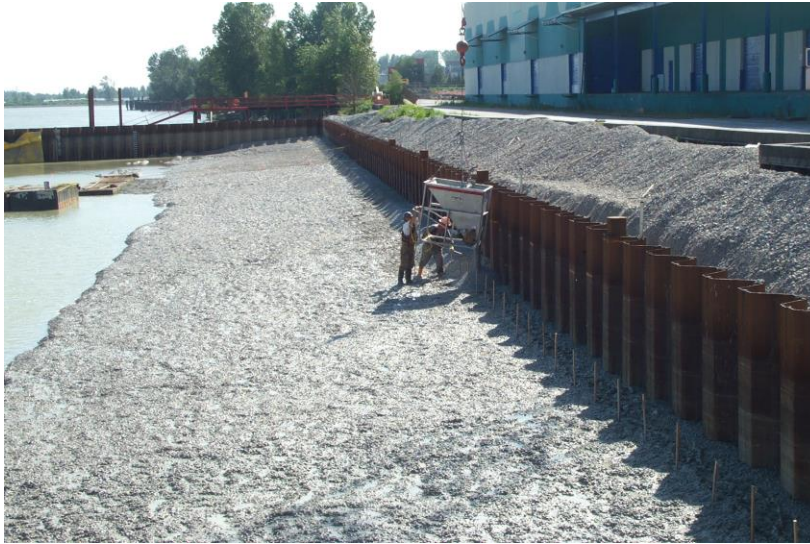
Photo #2: AquaBlok Placement Along Sheet Pile Wall
