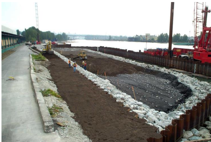
Photo #3: Installation of Marsh Topsoil for Wetland
